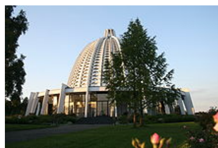
Bahá'í House of Worship, Langenhain, Germany
